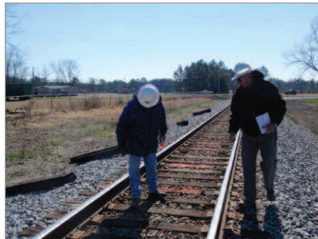
Terry Amburgey and Jim Watt mark ties for removal in 2010 just prior to the field trip.
