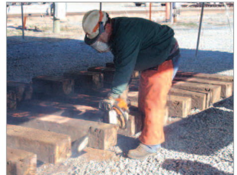
Ties being sectioned by NS personnel.
